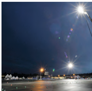
New stadium lights
